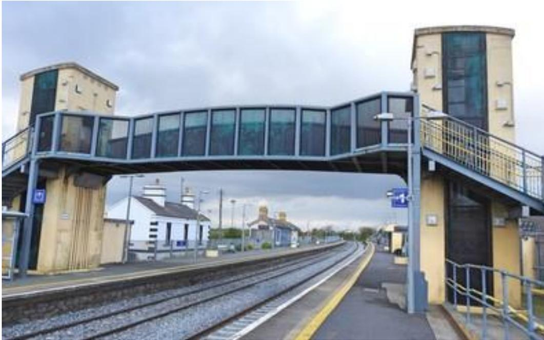
**Figure 2-31: Footbridge with stairs and lifts at both sides**
