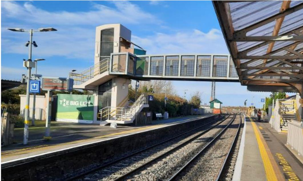
**Figure 2-18: Footbridge with stairs and lifts at both sides**
