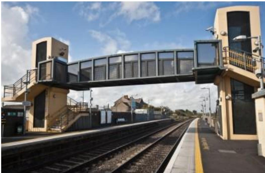
Figure 2-23: Footbridge with stairs and lifts at both platforms
