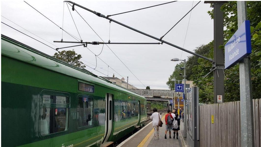
**Figure 5-9: Example of existing single-track cantilever at Malahide Station**
