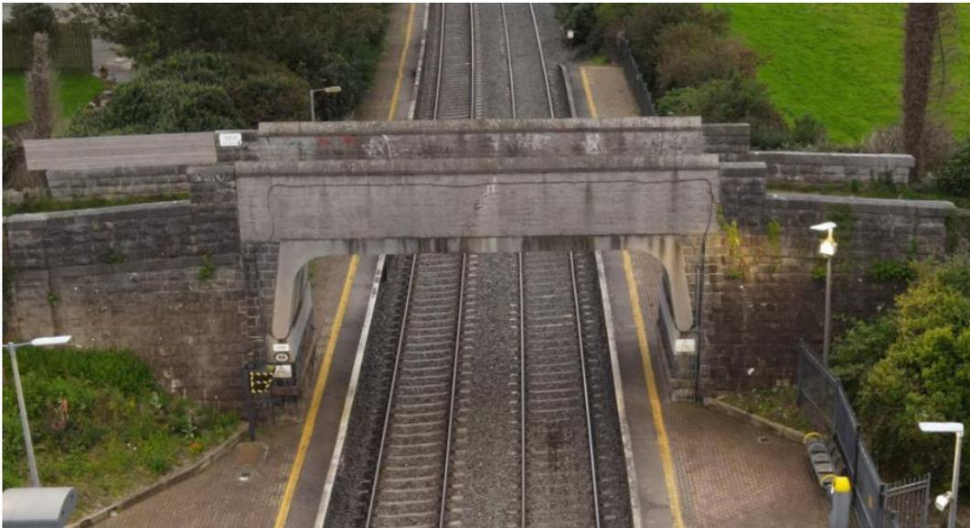
**Figure 5-21: Overbridge at Gormanston Station. Note the narrow passage under the bridge.**
