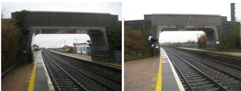
Figure 2-27: Overbridge with low clearance height at the south side of the platforms. Left to right: north elevation, south elevation (Source: Irish Rail)
