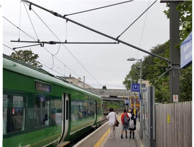
**Figure 2-2: Single track cantilever at Malahide Station**
