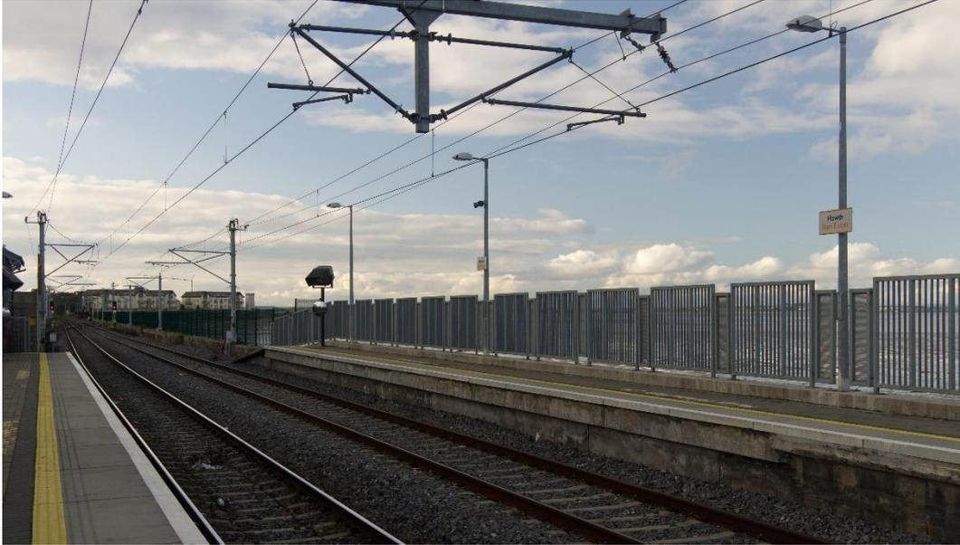
**Figure 5-11: Current two track cantilever at Howth Station**
