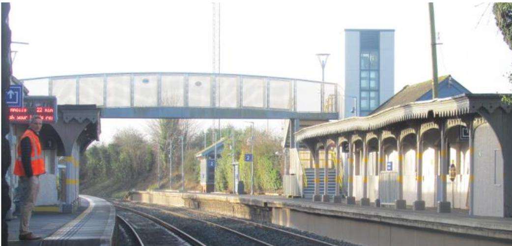
**Figure 2-14: Footbridge OBB38A at the north end of the platforms with lifts and stairs at both sides**
