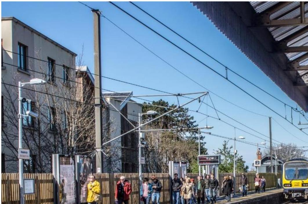
**Figure 5-10: Example of existing single-track cantilever at Malahide Station**
