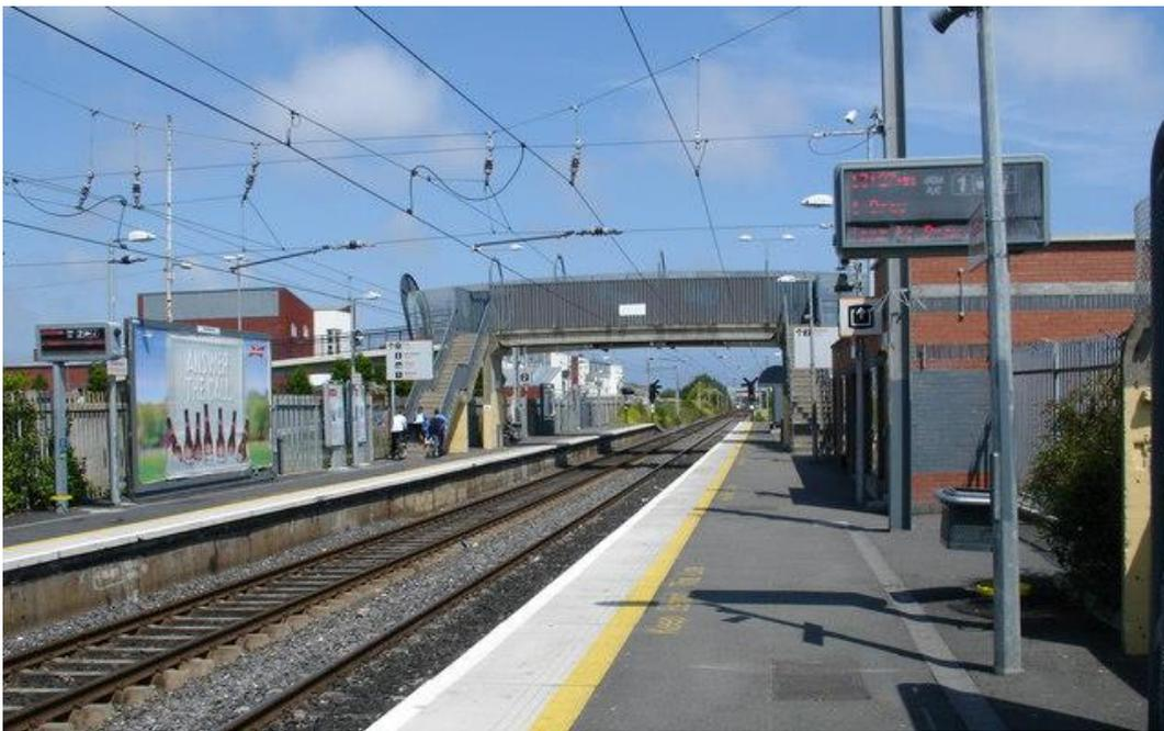
**Figure 5-12: Existing head span at Kilbarrack Station**
